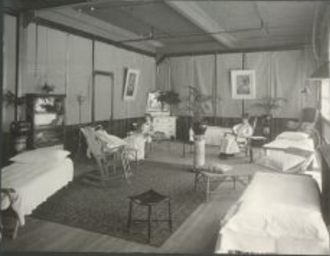
WOMEN'S REST ROOM
