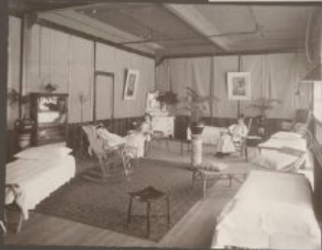
WOMEN'S REST ROOM
